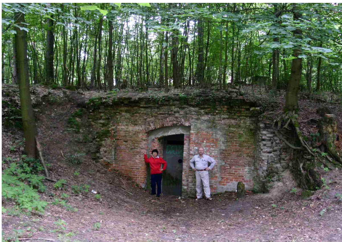
Fig. #D5(a): The exit from an underground tunnel. It is hidden in forest not far from Cieszków (i.e. around 8 km north from Milicz). The photograph taken in July 2004. In order to illustrate the size of this tunnel, at the exit gate stands myself (i.e. Dr Jan Pajak) and my wife . People used to say, that this tunnel originally was connected with the fortified castle in Milicz. But before the second world war a final part of it was separated from the rest by a wall, and utilised by a local distillery as a cellar for maturing alcohols. Presently this tunnel is established as bats reservation. The entrance to (or rather an exit from) it is locked permanently and inaccessible for the general public.
